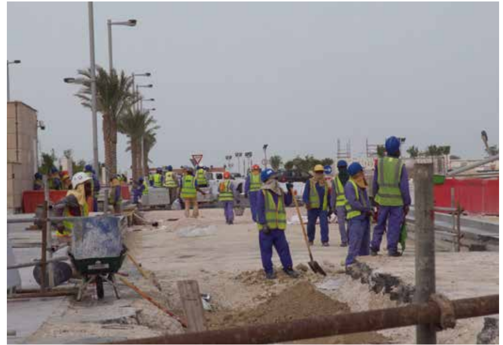
WM-Baustelle in Katar © Amnesty International
